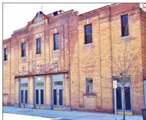
Colonial Theater undergoes major renovations.
